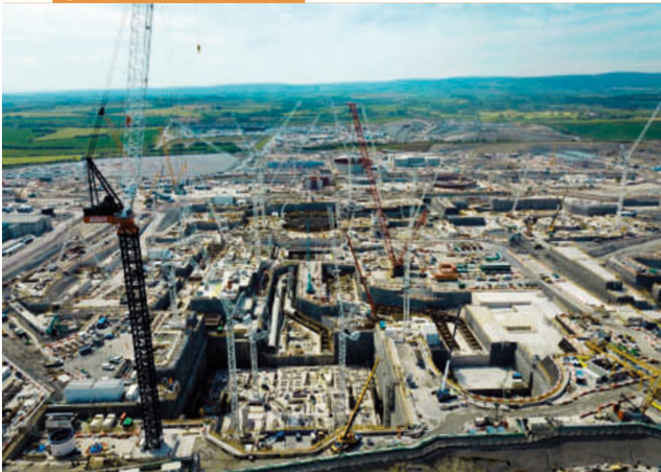
Figure 42 - The Hinkley Point C Construction Site
